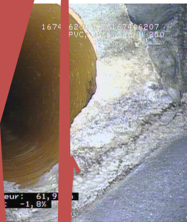
Infiltration calcaire
